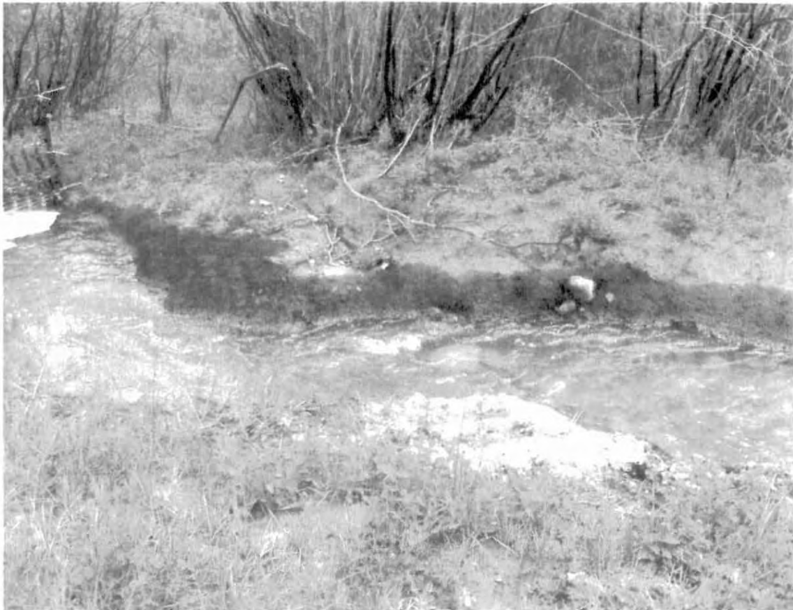
View to the east of the flowing stream at the north end of the planned excavation area. Note the padding in place (far left of photo) as countermeasure to the crude release. Crude 'staining' is also visible along the bank immediately above the water line.
