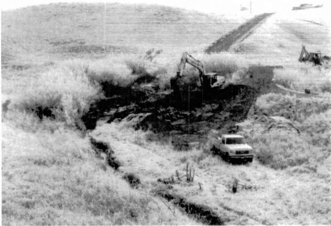
View to the south showing remediation activities. Photo taken: December 10, 2004
