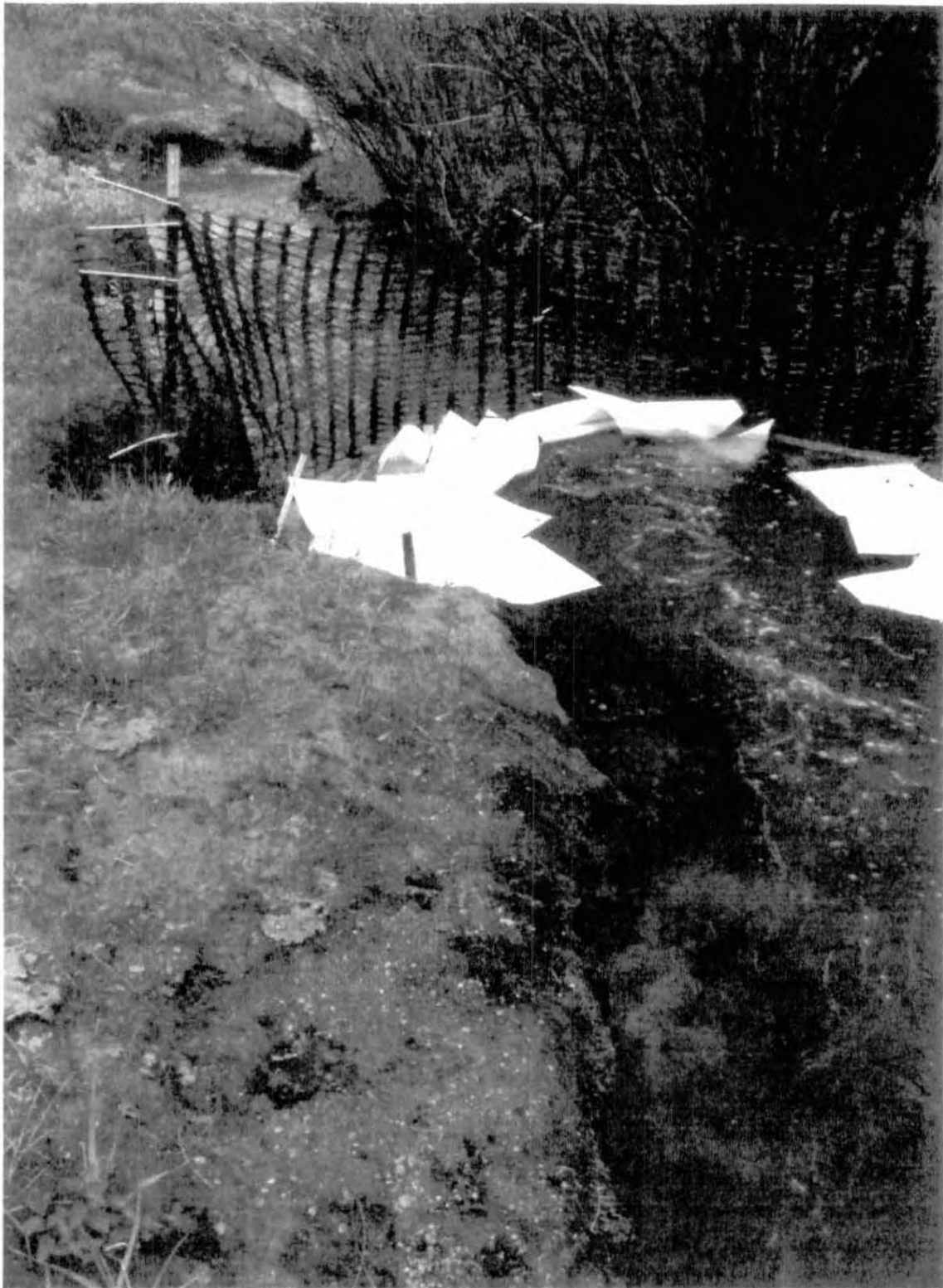
View to the north of the flowing stream at the north end of the planned excavation area. Note the padding in place as countermeasure to the crude release. Crude 'staining' is also visible along the bank immediately above the water line.
