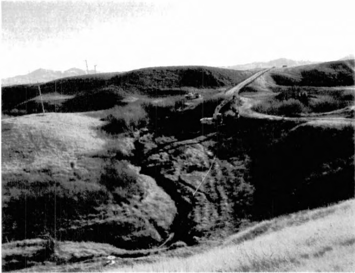
View to the south showing remediation activities. Photo taken: December 10, 2004
