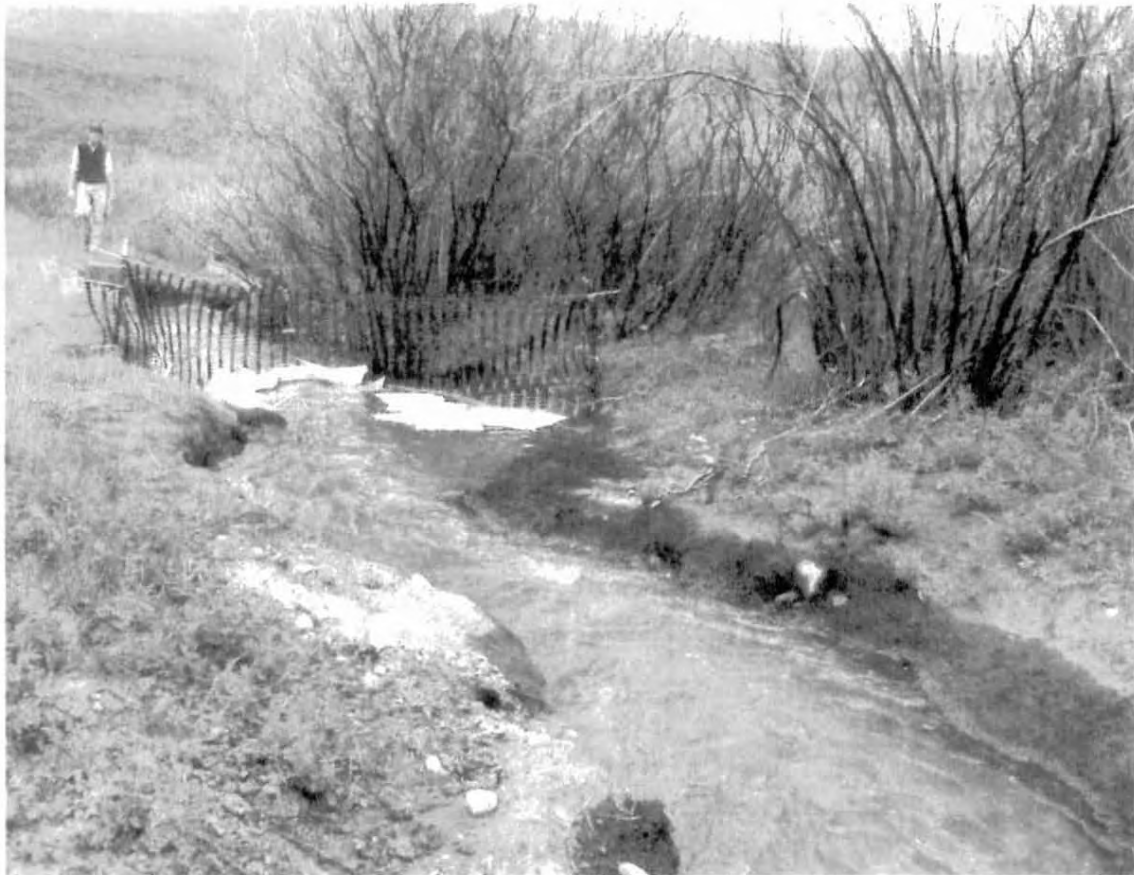
View to the north of the flowing stream at the north end of the planned excavation area. Note the padding in place as countermeasure to the crude release. Crude 'staining' is also visible along the bank immediately above the water line.
