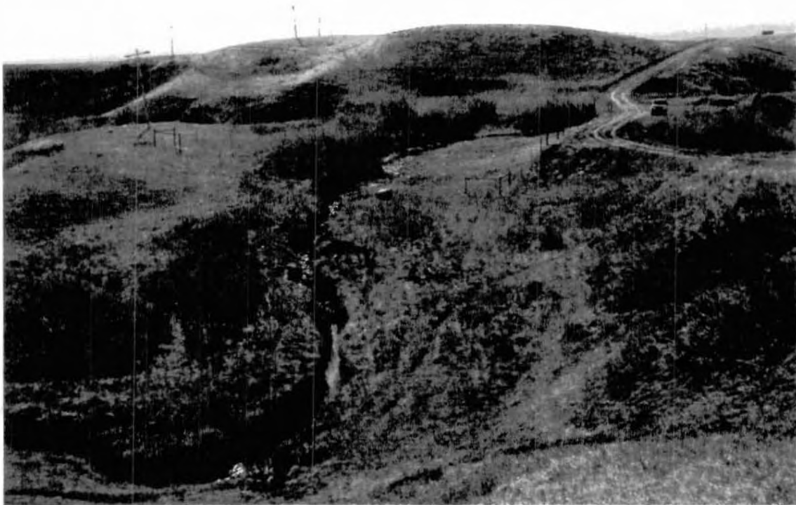
View to the south showing remediation area. Note that vegetation is beginning to fill in where topsoils were replaced after the excavation and bank reconstruction.
