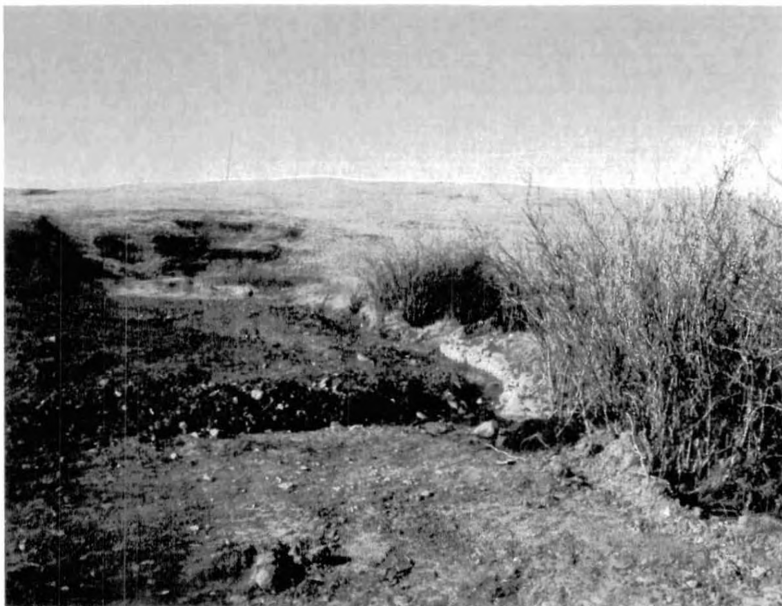
View to the north showing the pre-vegetation state following bank reconstruction. Sandbags on the east bank of the stream were placed in March 2005.
